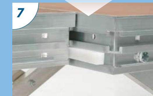
Plastic rails reduced movement of stage platform
